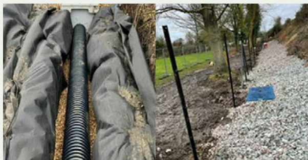
Catchpit and pipe runs and final re-instatement
