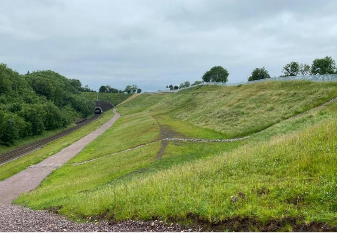
Figure 14: Harbury cutting following works.
