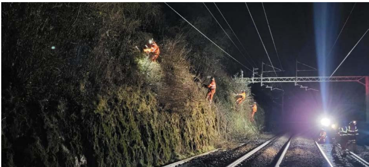
Figure 7: Tring Cutting Vegetation Management in Action
