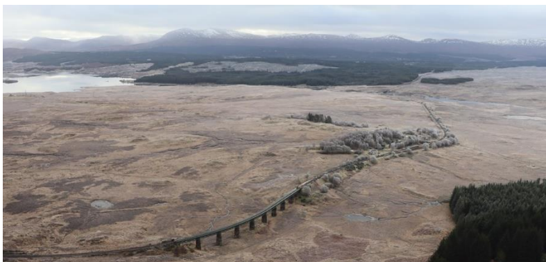
Figure 4: A section of the West Highland Line located in Rannoch
