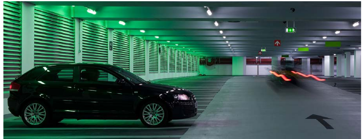
Image 4.20: Covered parking garage - Coloured light at the perimeter of the space assists wayfinding whilst white lighting on the driving lane provides good levels of illuminance for all user
