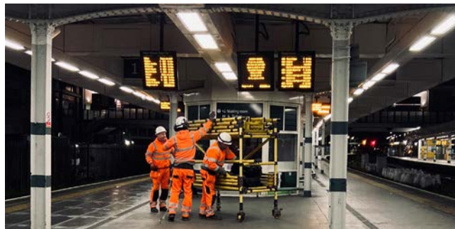
Image 7.7: Use of mobile scaffold tower for maintenance of platform lighting.
