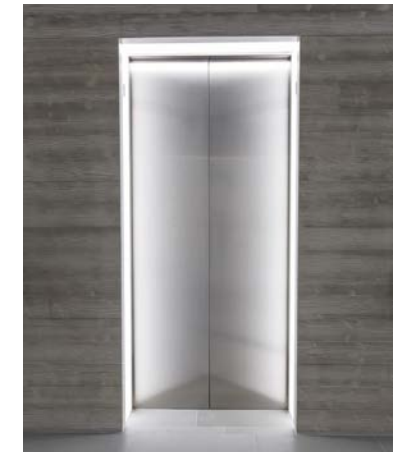
Image 4.40: Lighting detail within the lift's alcove. Unibox ,UK
