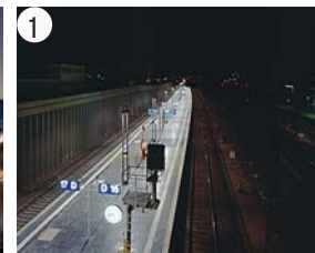
Image 4.57: Asymmetric lanterns aligned with centreline of island platform create shadow-free illumination up to platform edge
