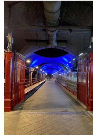
Image 4.53: Leeds Station Wall mounted LED uplights illuminate the vaulted ceiling creating visual interest and assisting passenger orientation..
