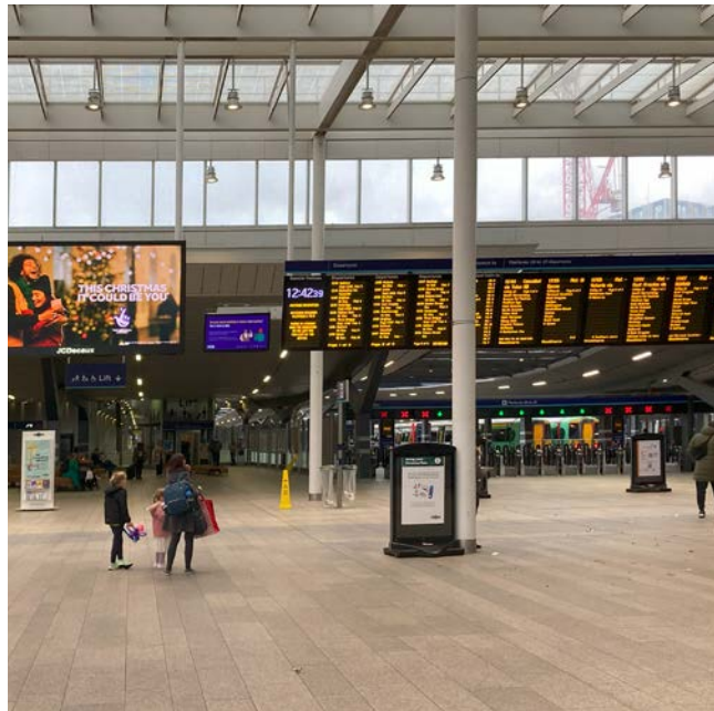
Image 2.5: London Bridge Concourse area during daytime. A translucent frit on the glazed roof creates diffused daylight during the day providing ambient illumination for the circulation spaces.
