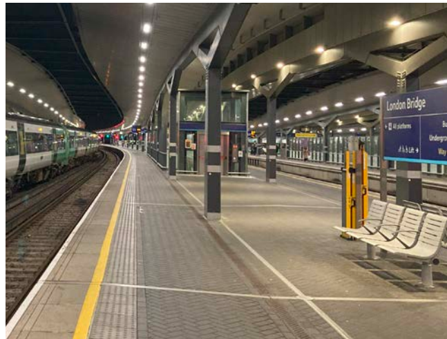
Image 2.11: London Bridge - Train Platform Platform edge lighting avoids high contrast and shadows
