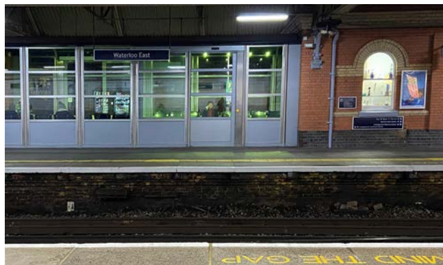
Image 4.70: Enclosed waiting room with clear glazing enables passengers to see in and out of the space.
