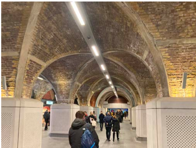
Image 2.10: London Bridge - Undercroft Suspended multi-service lighting trough supports wayfinding
