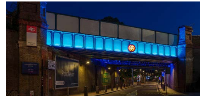
Image 4.48: Wandsworth Town Station Rail Bridge Cast iron panels illuminated with linear RGB lighting
