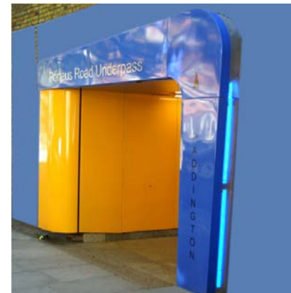
Image 8.27: Blue Tunnel Portal
