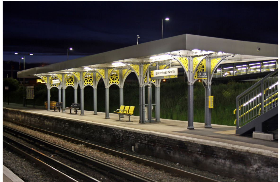
Image 8.30: Birkenhead North Station The colour scheme and the lighting design combine to create an attractive and welcoming platform environment at night.
