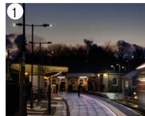
Image 4.56: Pole mounted luminaires aligned with centreline of island platform create shadow-free illumination up to platform edge
