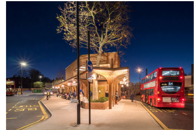
Image 4.11: West Croydon Bus Station. Direct/Indirect pendant downlights suspended below canopy with translucent ceiling panels providing soft upright to station signage located above canopy
