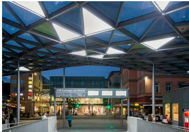
Image 4.10: Esslingen ZOB, German. Diffuse LED light panels integrated with canopy design provide ambient light to bus station
