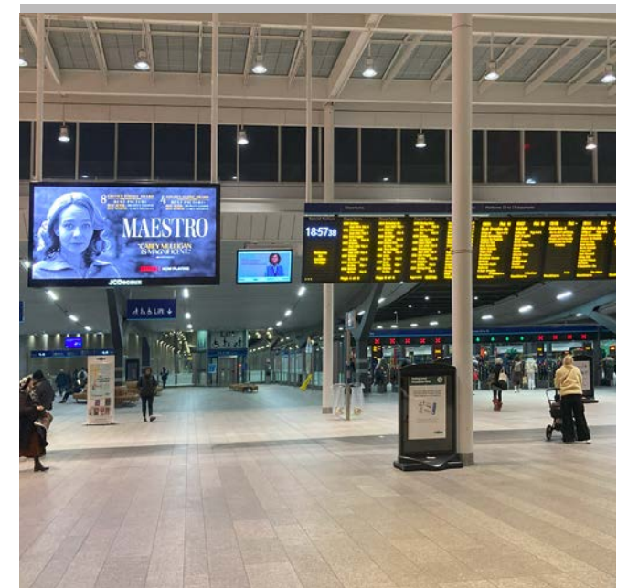
Image 2.6: London Bridge Concourse area after dark. A variety of luminaire types and lighting elements create a different experience at night. The windows are dark but the translucent frit on the glazed roof reflects light back onto the circulation space below. The glazed roof appears more opaque at night than it does during the day.
