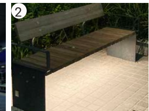
Image 4.63: Additional accent lighting concealed under benches can provide enhanced levels of illuminance to promote passenger comfort
