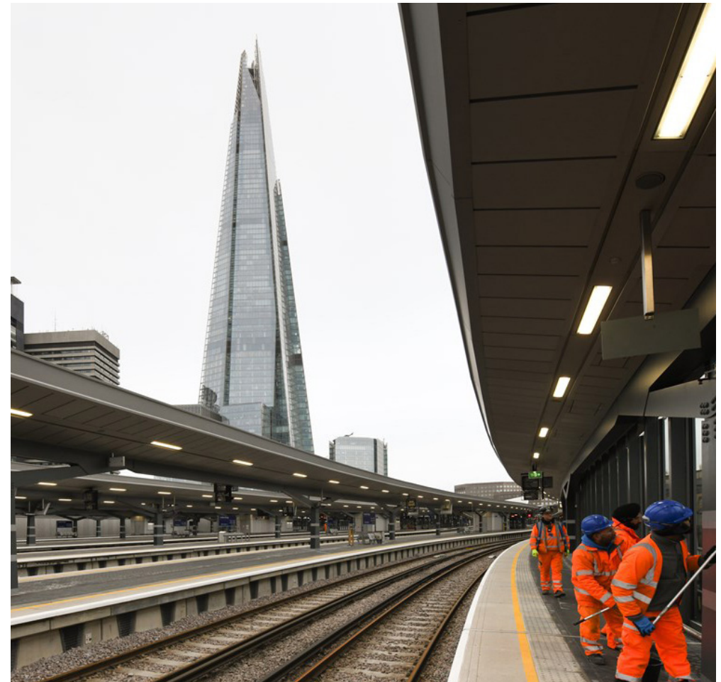
Image 7.5: London Bridge platform under construction
