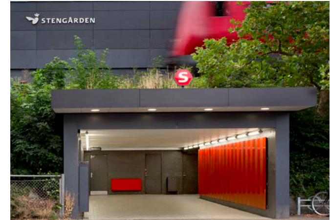
Image 4.54: Stengården Station - Underpass Continuously mounted tubular prismatic luminaires highlight ceilings and wall surfaces creating a sense of spaciousness. Bright coloured cladding panels are part of the station branding.
