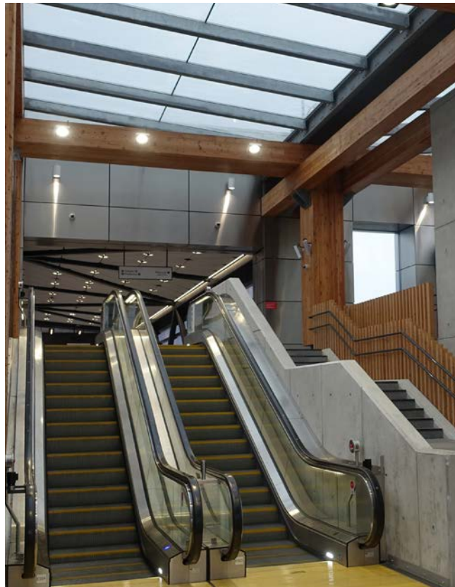
Image 3.3: Brent Cross West Station Concourse with diffused ceiling openings allowing daylight in the space
