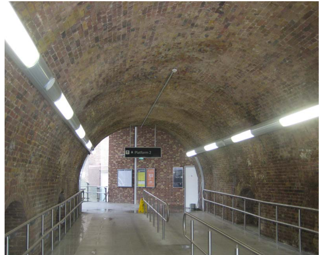
Image 7.3: Typical Cable Management System (CMS) railway arch underpass at street level.
