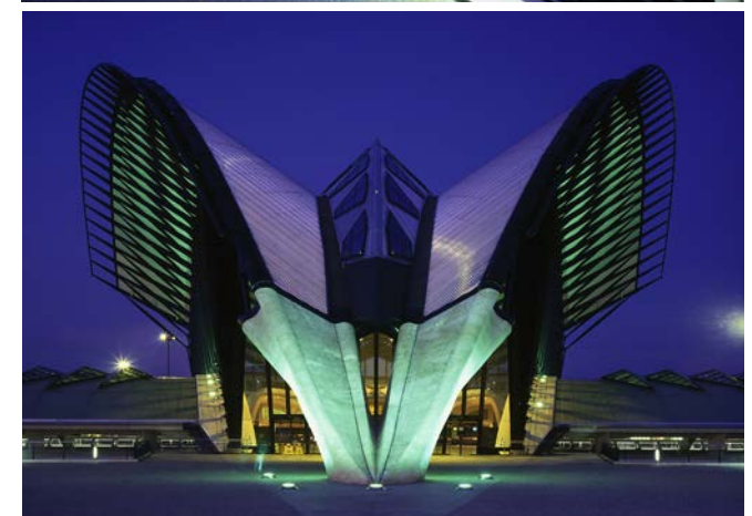
Images 1.3 and 1.4: Lyon-Saint Exupéry Airport Railway Station The sculptural form of the station canopy is transformed at night with indirect lighting to create an iconic ‘gateway to the city at night’.
