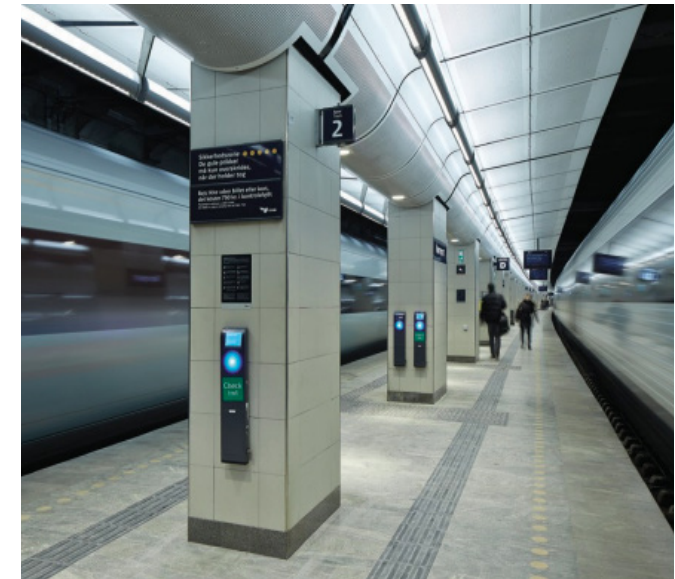
Image 8.7: The refurbished platforms at Nørreport Station. Direct/Indirect lighting creates a sense of spaciousness, an elevated ceiling and more comfortable environment for passengers.
