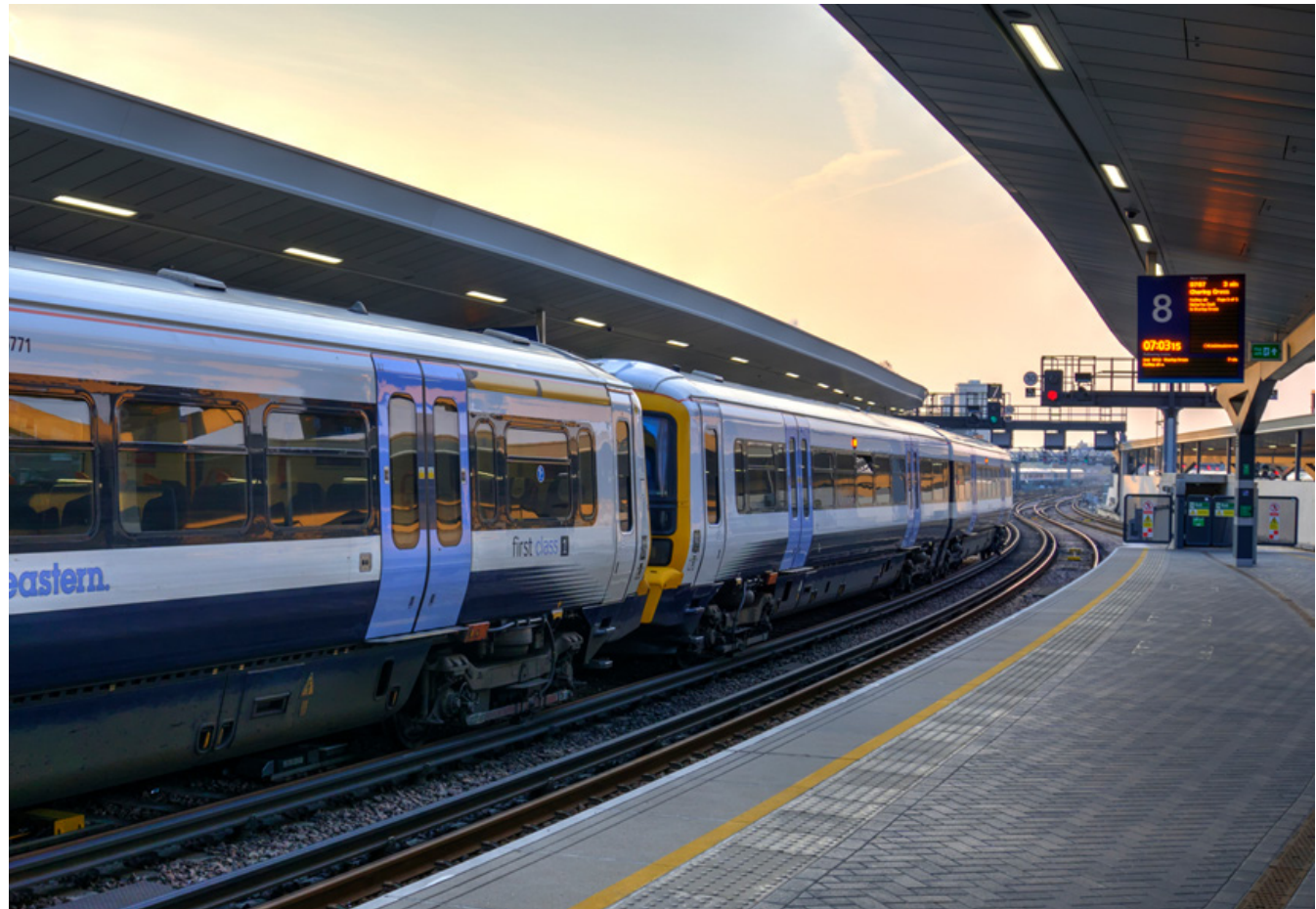
Image 1.6: London Bridge Station Multi-service channels with Cable Management System (CMS), Closed Circuit Television (CCTV) and lighting flush recessed into canopy soffit panels
