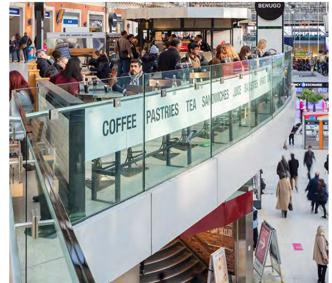
Image 2.66 London Waterloo Station- Toughened Glass Balustrades
