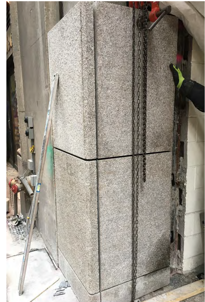
Image 2.25 Installation of Granite cladding
