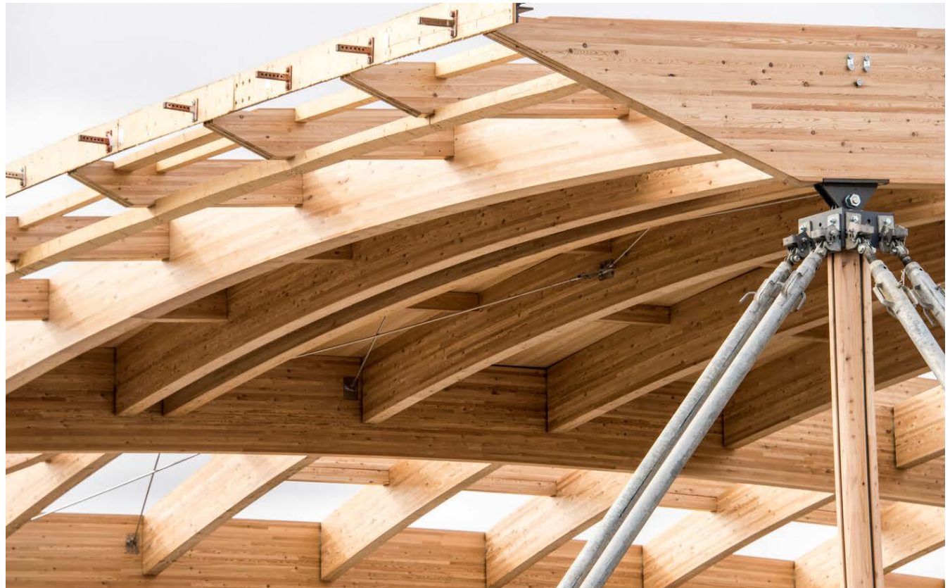
Image 1.50 Abbey Wood Station - Larch and Spruce Glue-laminated timber roof and soffit
