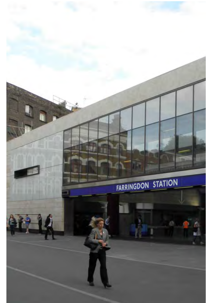
Image 2.34 Farringdon Station - Stone rainscreen cladding
