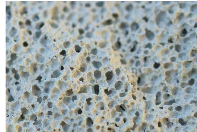
Image 1.13 RAAC - Reinforced Autoclaved Aerated Concrete
