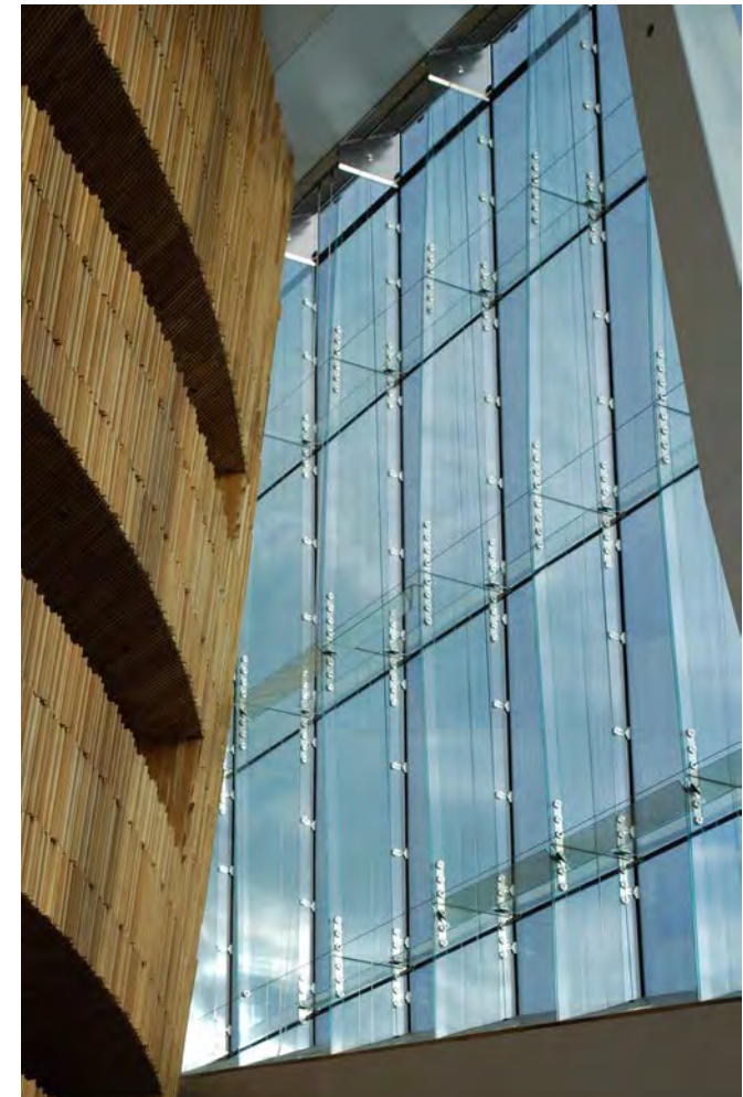
Image 2.68 Structural Glass Curtain Walling
