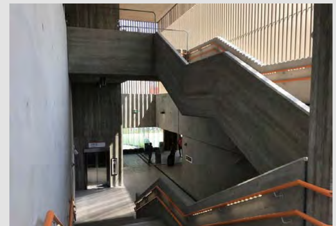
Image C.5 Hackney Wick station cast concrete stairs viewed from top and intermediate landings
