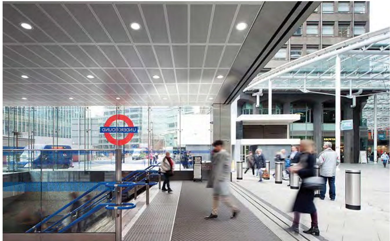
Image 1.51 SIDOS compliant ceiling at London Underground station entrance
