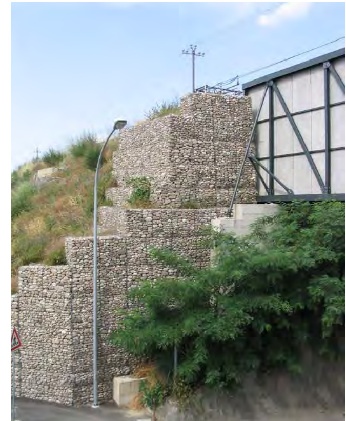
Image 2.33 Retaining wall constructed with gabions
