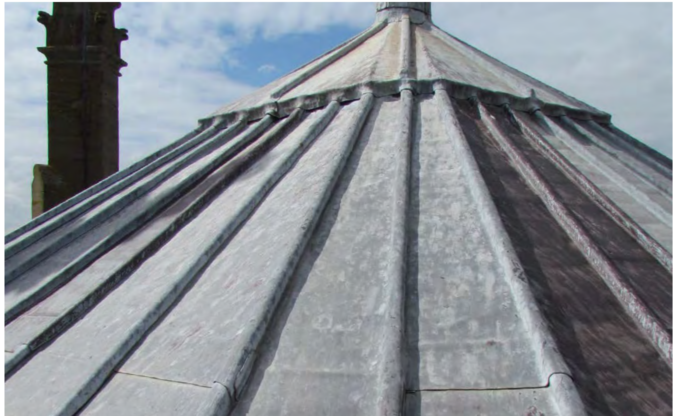
Image 2.56 Traditional lead roof at St. Laurence's Church, Ludlow
