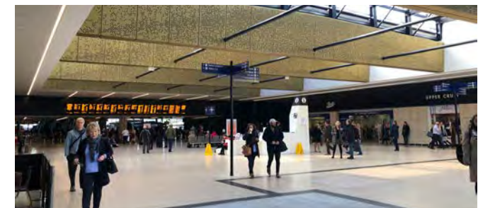
Image 1.25 Leeds City Station concourse with retail
