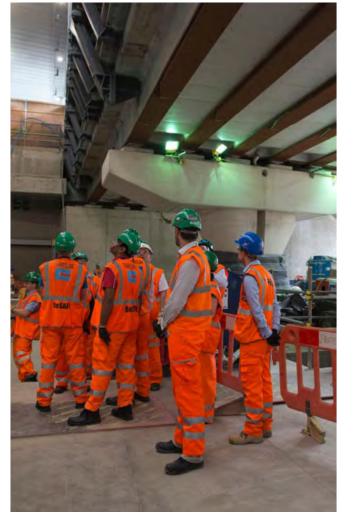
Image 4.2 London Bridge station refurbishment during construction
