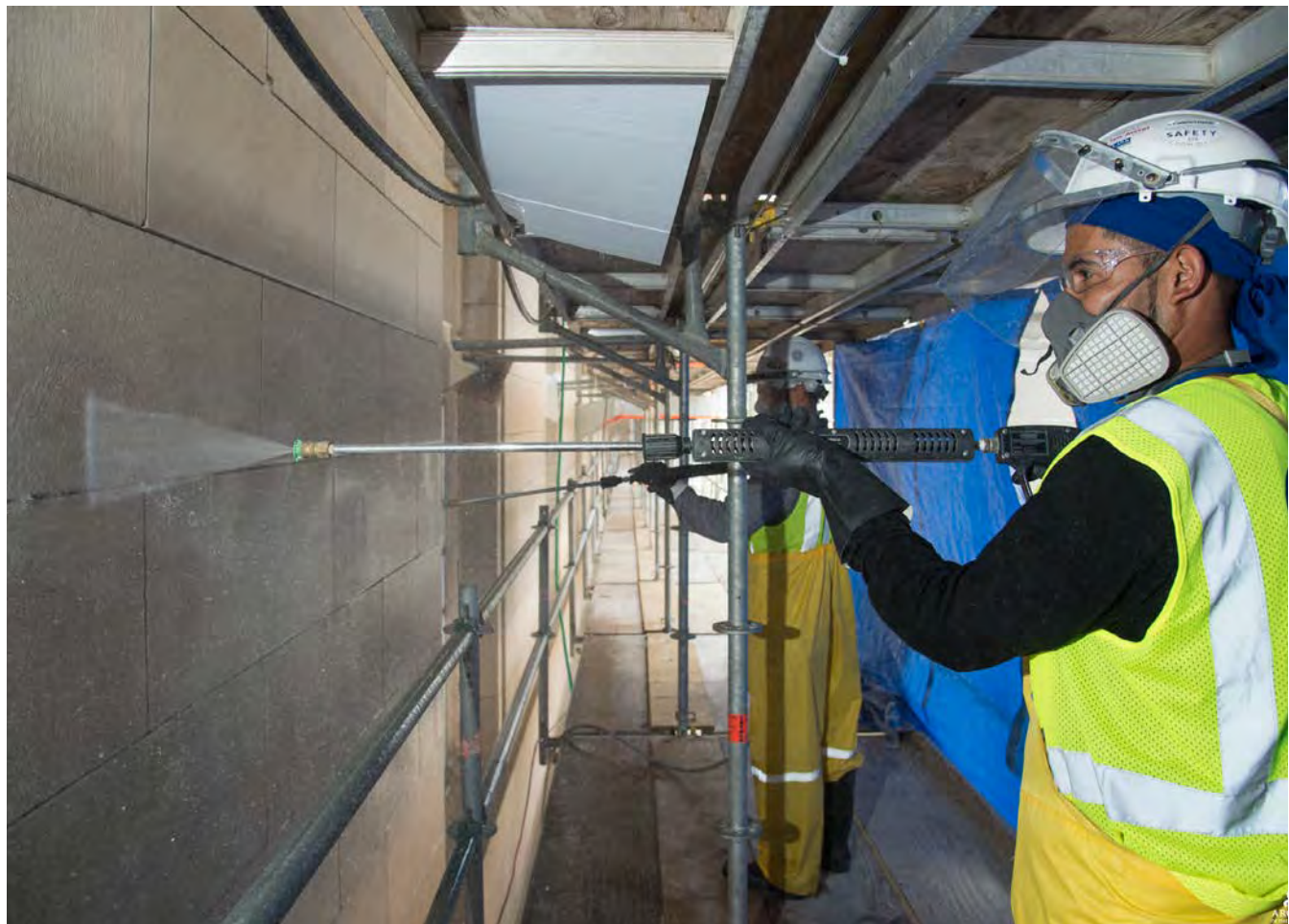
Image 2.35 Cleaning and maintenance of natural stone facade
