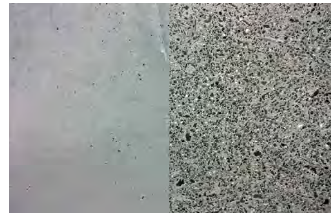
Image 2.46 Smooth concrete surface next to acid etched finish
