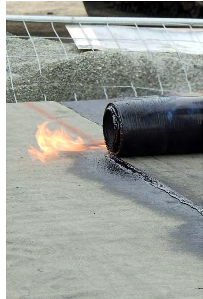
Image 2.73 Welded application of reinforced bitumen membrane
