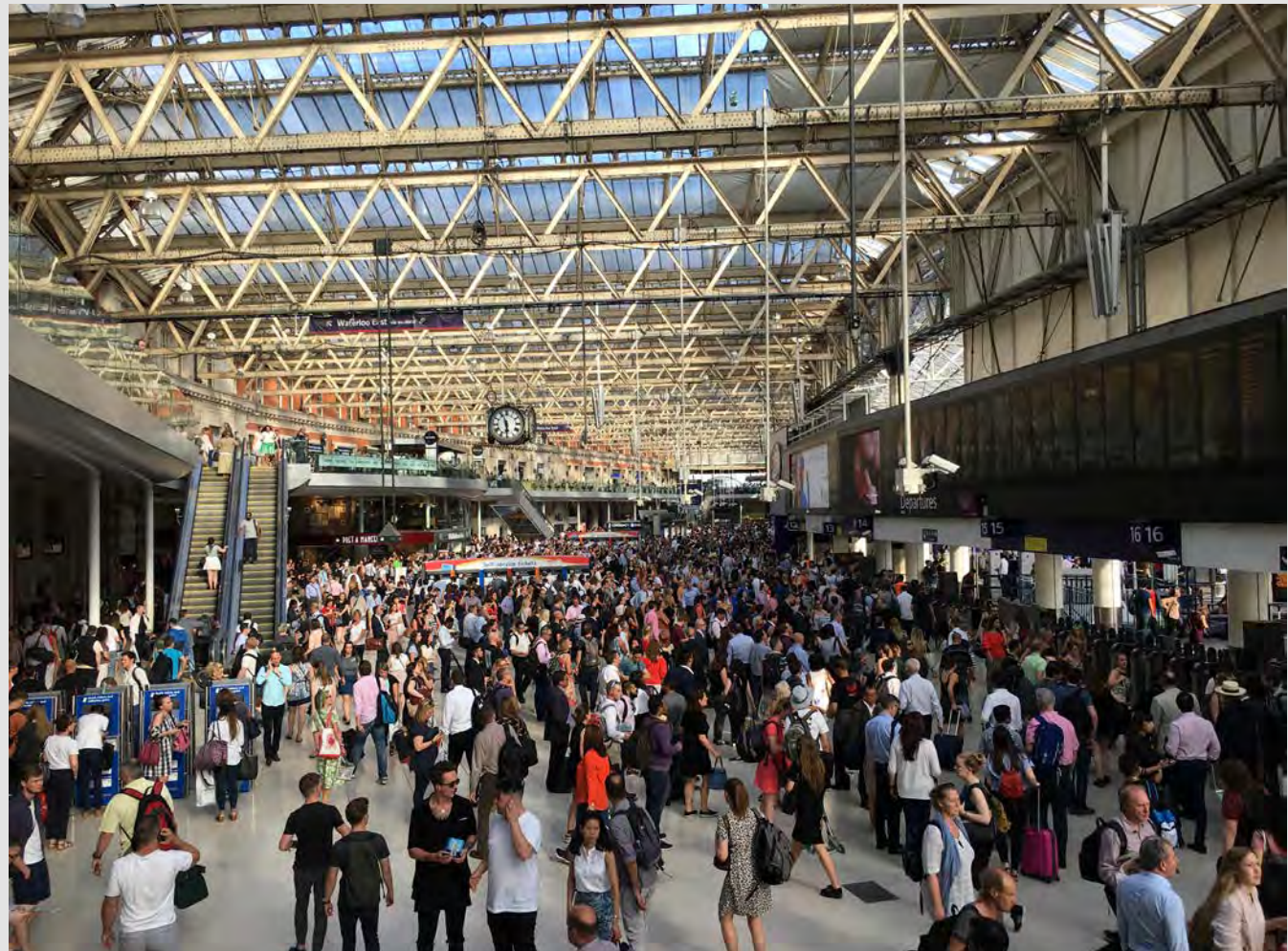
Image C.2 Waterloo Station roof viewed from the concourse
