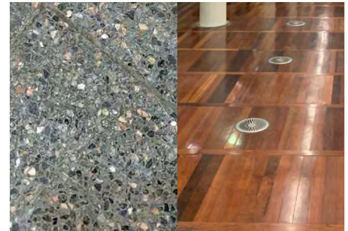
Image 1.17 Unique terrazzo and parquet jatoba flooring at St Pancras International
