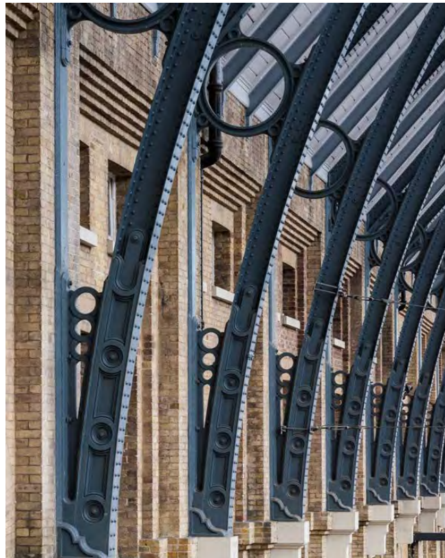
Image 1.3 Kings Cross Station - Historic Train Shed Structure
