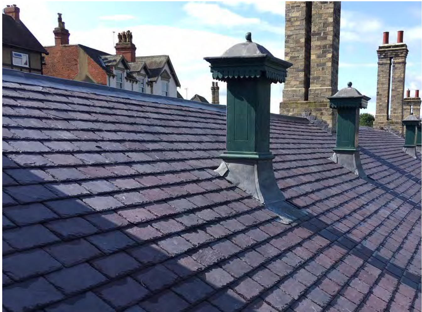
Image 2.28 New roof slates at Knaresborough station
