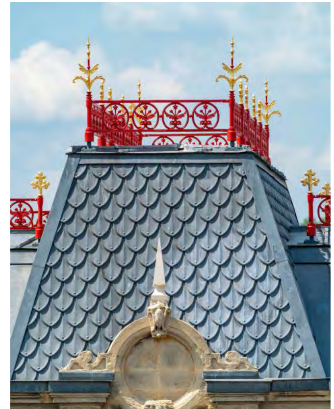
Image 1.53 Peckham Rye - Restored Station Roof
