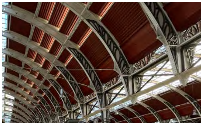
Image 1.46 London Paddington - Train Shed Roof
