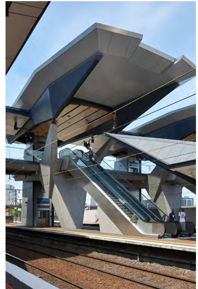
Image 2.54 North Melbourne Station - Stainless Steel
