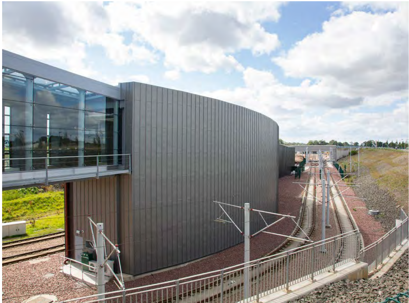
Image 2.61 Zinc cladding - Edinburgh Gateway station
