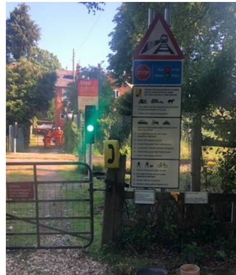
Figure 4-6 Interfaced Overlay at Smiths crossing (Wessex)
