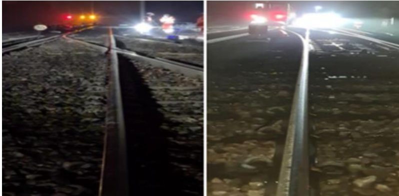
Fig 8-4 Improved alignment at Surbiton Junction post work
