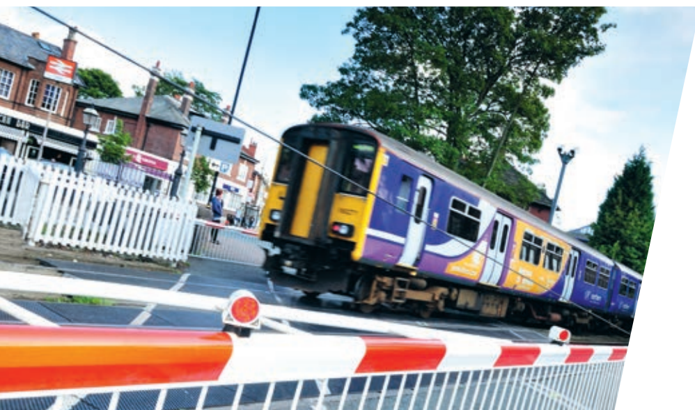
Above: Full barrier level crossing.
