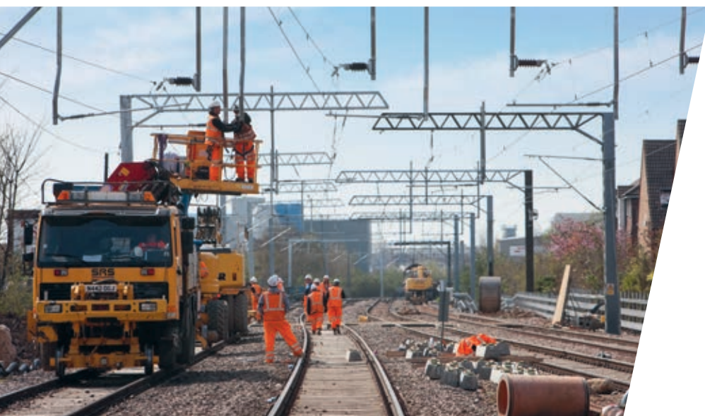
Above: North London line maintenance.
